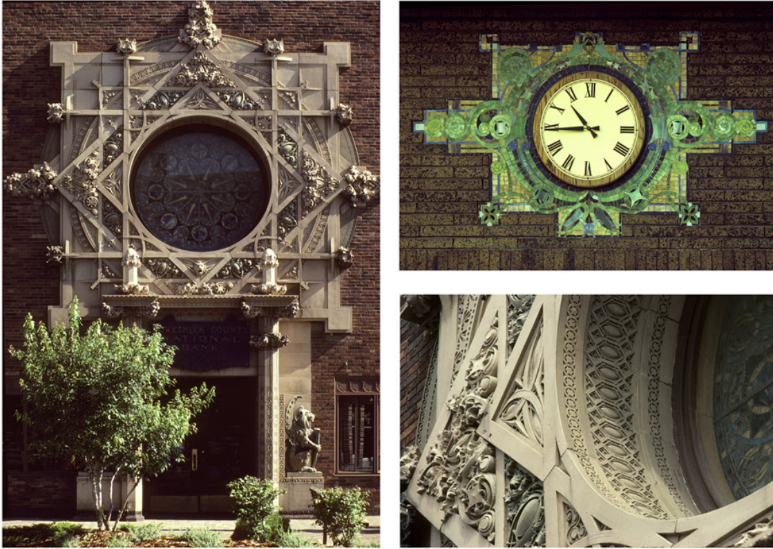
Louis H. Sullivan (US, 1856-1924), Merchants National Bank (Brenton National Bank of Poweshiek County), Grinnell, Iowa, 1899. [L] View of main (south) entrance; [TR] South wall clock above main entrance showing glazed brick and glass mosaic; [BR] Detail of glazed terracotta cartouche surrounding the oculus above the main entrance. Among the finest of Sullivan's "jewel-box" Midwestern bank buildings, the Merchants National Bank was declared a National Historic Landmark in 1976. Photographs by Philip Larson.
