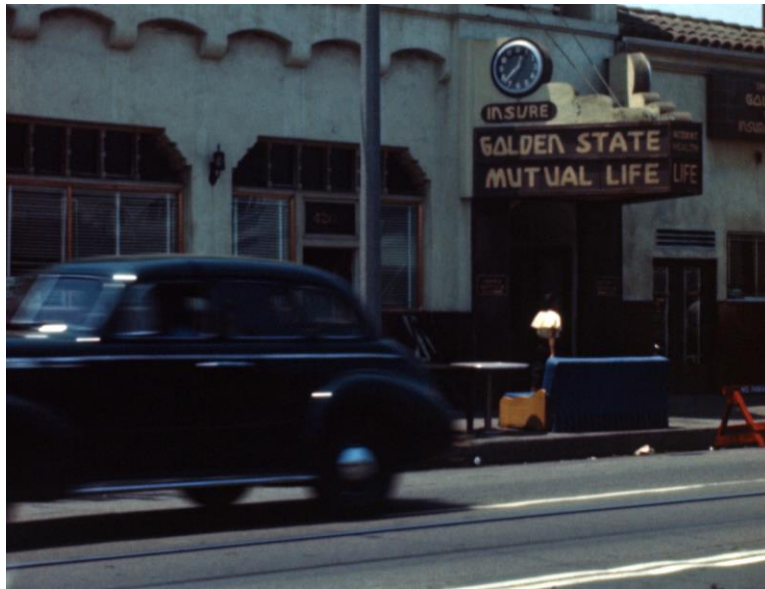
Home Office on Central Avenue.
