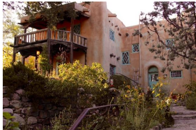
Figure 12: Witter Bynner House, Old Santa Fe Trail, Santa Fe, New Mexico (photographer: Audra Bellmore).
